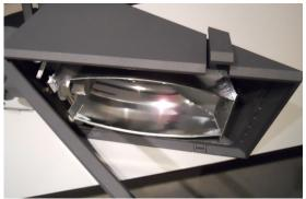
Lens cover frame will swing down after latches unclip
